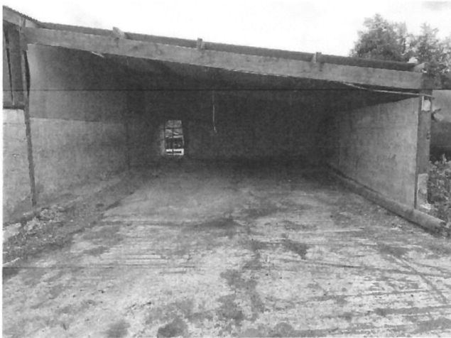
Shed in the process of being demolished
